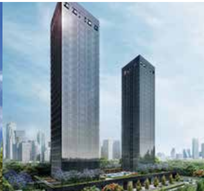
Trump Towers Pune India
