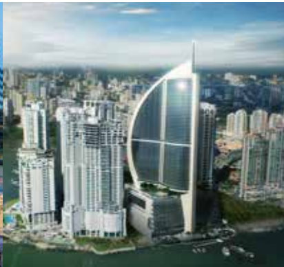
Trump International Hotel & Tower Panama City, Panama
