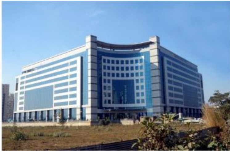
BESTECH BUSINESS TOWER SOHNA ROAD
