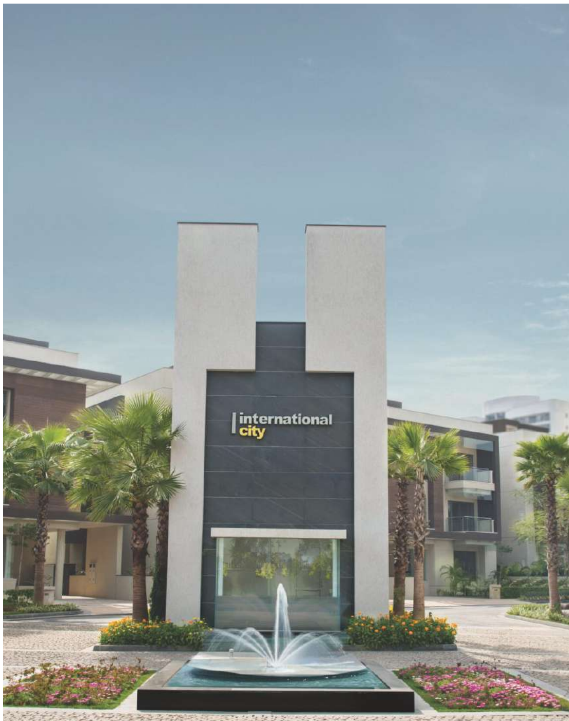
ACTUAL IMAGE OF THE BLOCK B ENTRANCE
