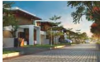
SOBHA Silver Estate, Thrissur
