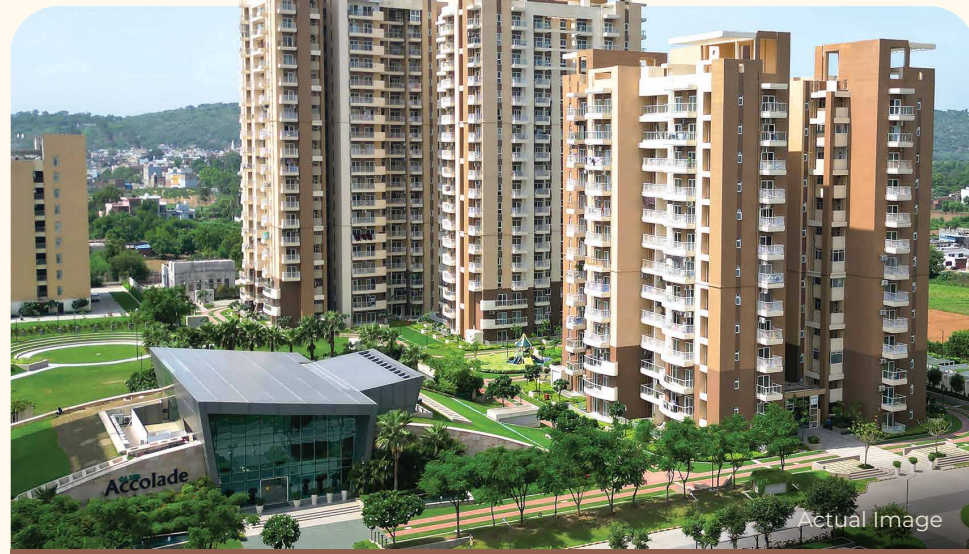
Eldeco Accolade, Sec 2, Sohna Road, Sohna
