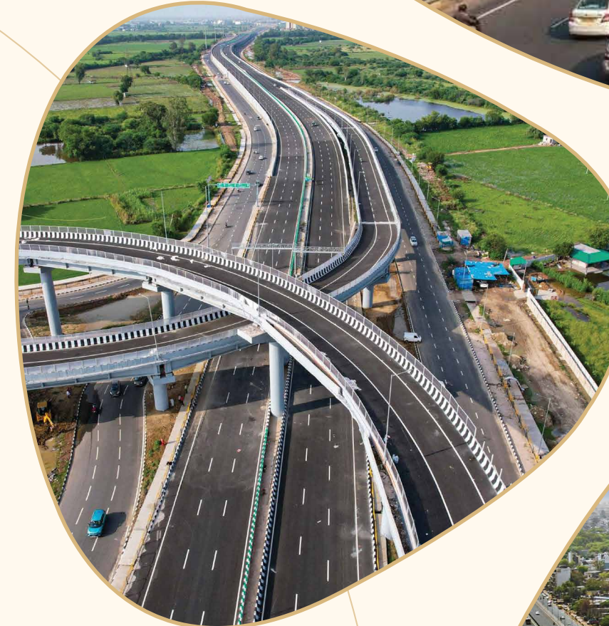
Dwarka Expressway 5 km
